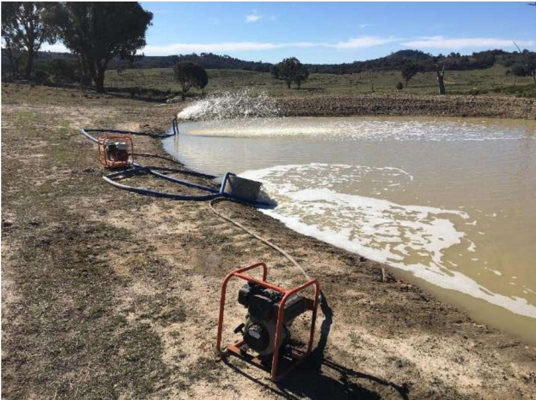
**Figure 8:** Post rain water management (manual flocking in process utilising floc blocks)
