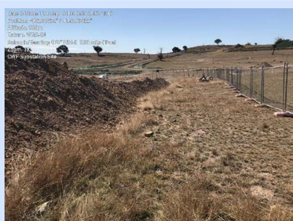
Photo 10. The topsoil bund at the top of the site directing clean water away.
