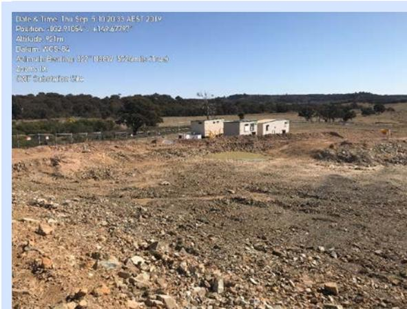
Photo 1. Water trapped in a low point of the excavation near the site offices.
