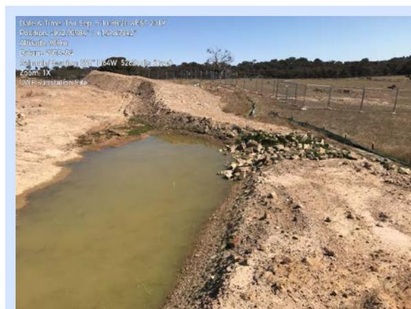
Photo 6. An overview of the sediment trap with rock lined spillway.
