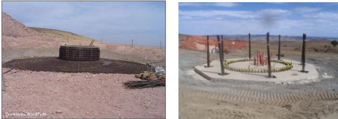
**Image 2: Typical gravity (left) and rock anchor (right) footings**
