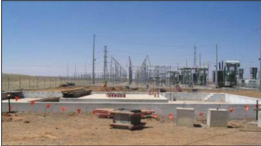
**Image 10: Transformer foundation (foreground) and electrical substation and switchgear infrastructure (background).**
