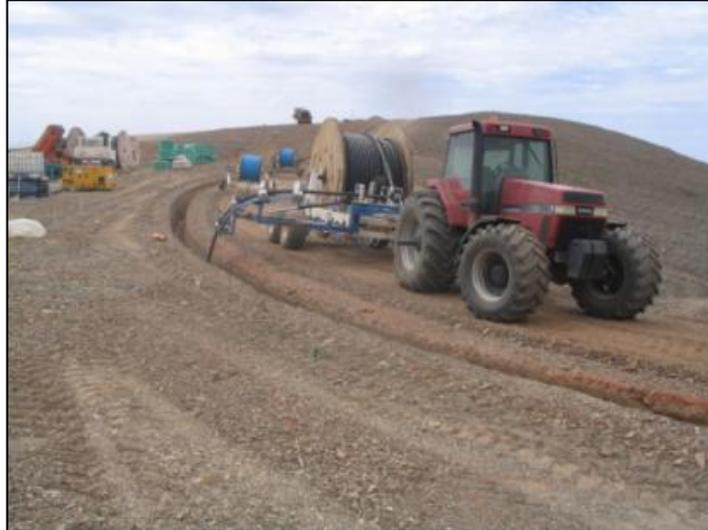
**Image 7: Laying underground electrical cable within the road network**
