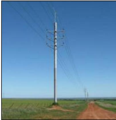
**Image 6: Typical overhead line construction that could be implemented in this proposal**
