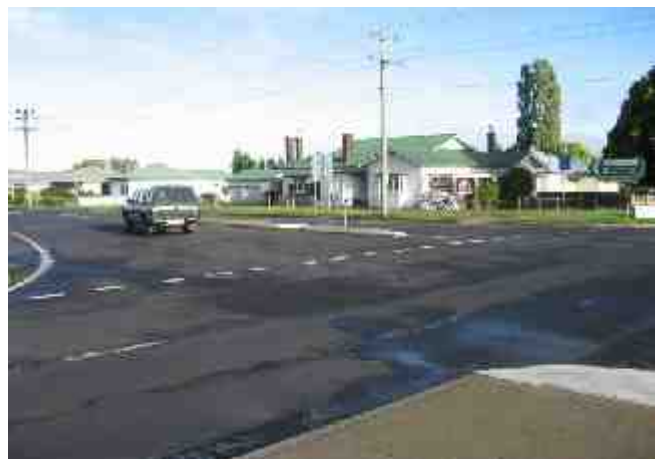
PLATE 6 Junction Gwydir & New England Highways looking West.
