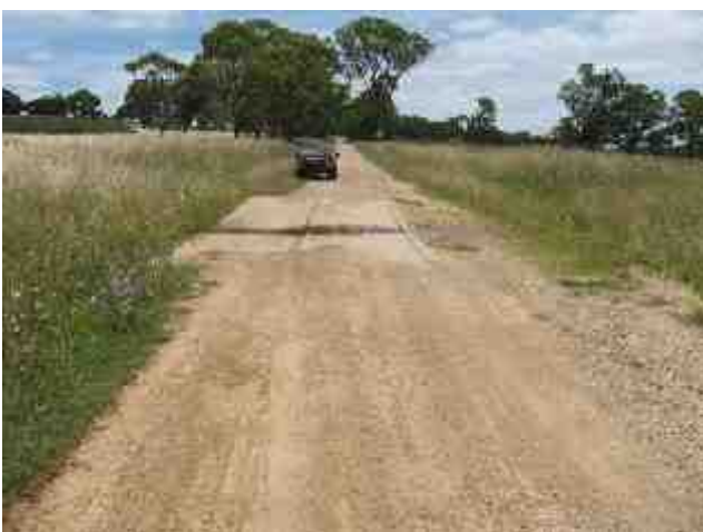
PLATE 41 Waterloo Rd, causeway at 14.80 km.
