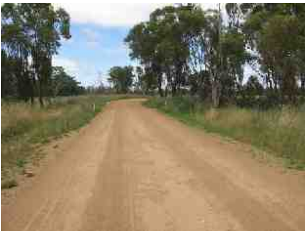
PLATE 21 Waterloo Road at 5.6 km.
