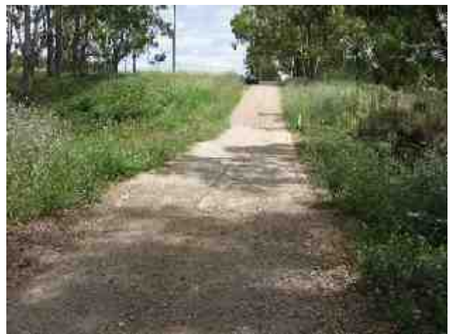
PLATE 30 Waterloo Rd, causeway at 9.5 km.
