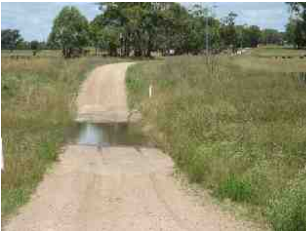
PLATE 45 Waterloo Road, causeway at 16.8 km.
