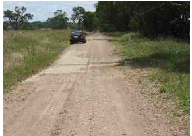
PLATE 44 Waterloo Road, causeway at 15.8 km.
