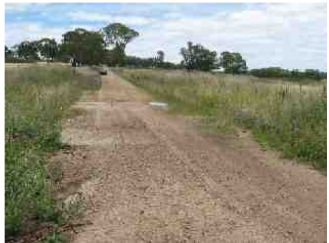
PLATE 40 Waterloo Rd, causeway at 14.75 km.
