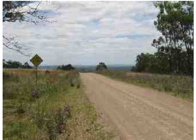
PLATE 50 Waterloo Road, warning sign at 19.6 km.
