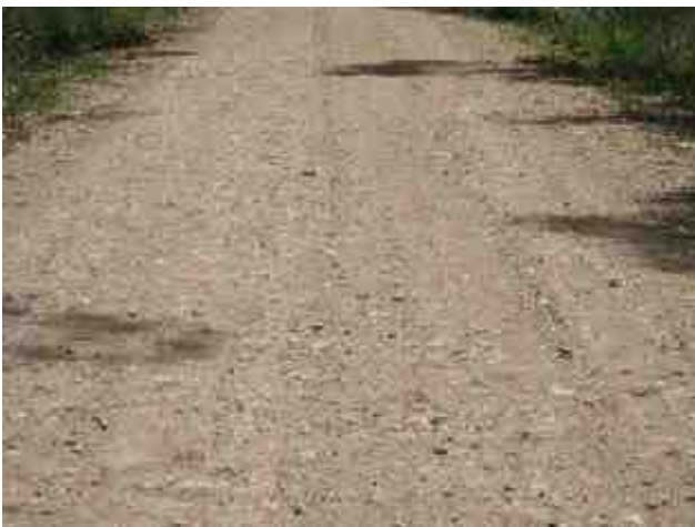
PLATE 27 Waterloo Road, surface at 8.2 km.
