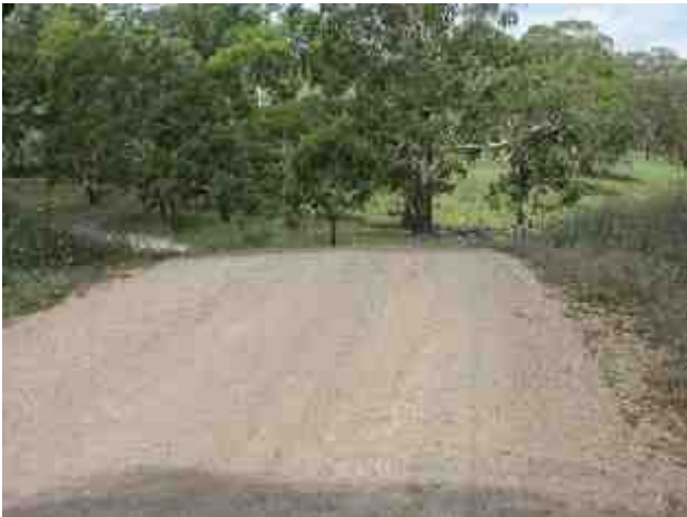
PLATE 49 Waterloo Road, Access at 18.5 km looking East.
