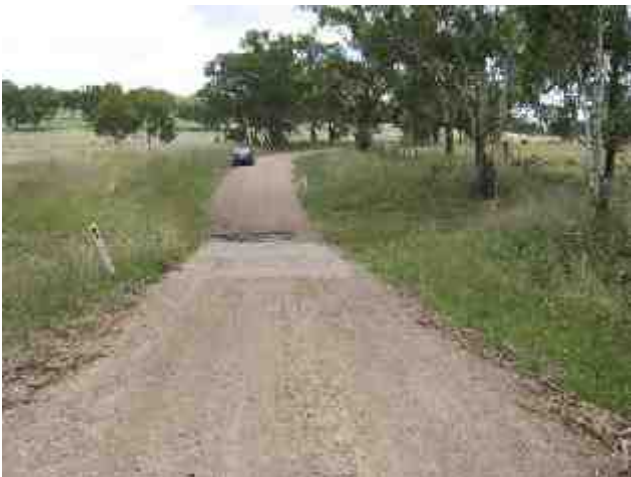
PLATE 39 Waterloo Road, causeway at 13.3 km.
