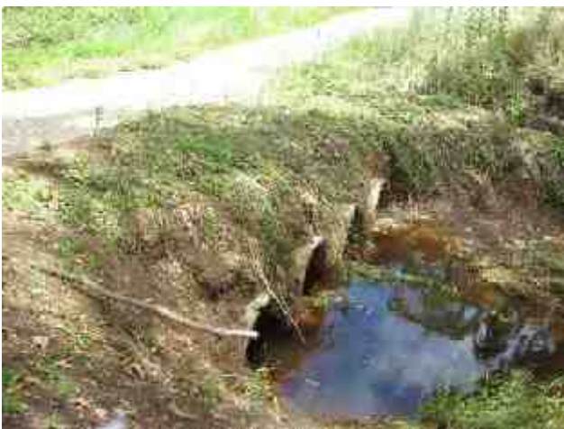
PLATE 29 Waterloo Rd, causeway at 9.5 km.
