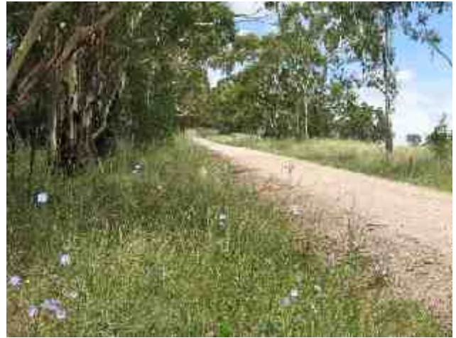
PLATE 26 Waterloo Road, Access at 7.8 km looking West.
